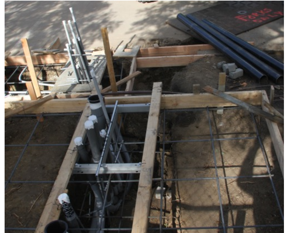
EV charging station installation construction
