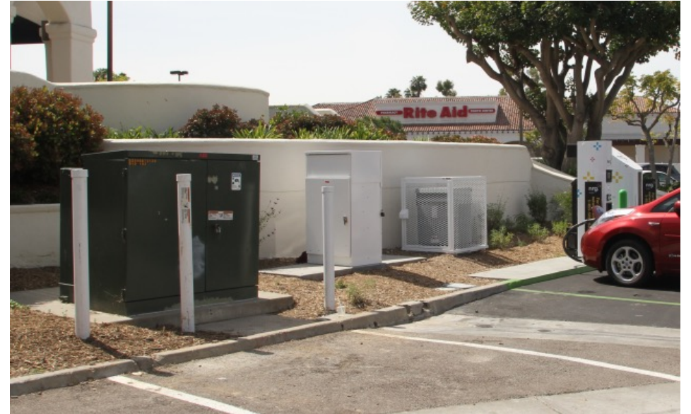
Benefit: Transformer & Meter Pedestal Close to Chargers
